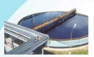
Known as a clarifier, is a circular tank in a sewage treatment plant (STP) that separates treated water from biomass. The Secondary Sedimentation Tanks are spherical tanks with motorized scum and sludge collectors that rotate. Spray systems for scum removal and odour control, as well as pumps for tank drainage, are examples of auxiliary systems.
